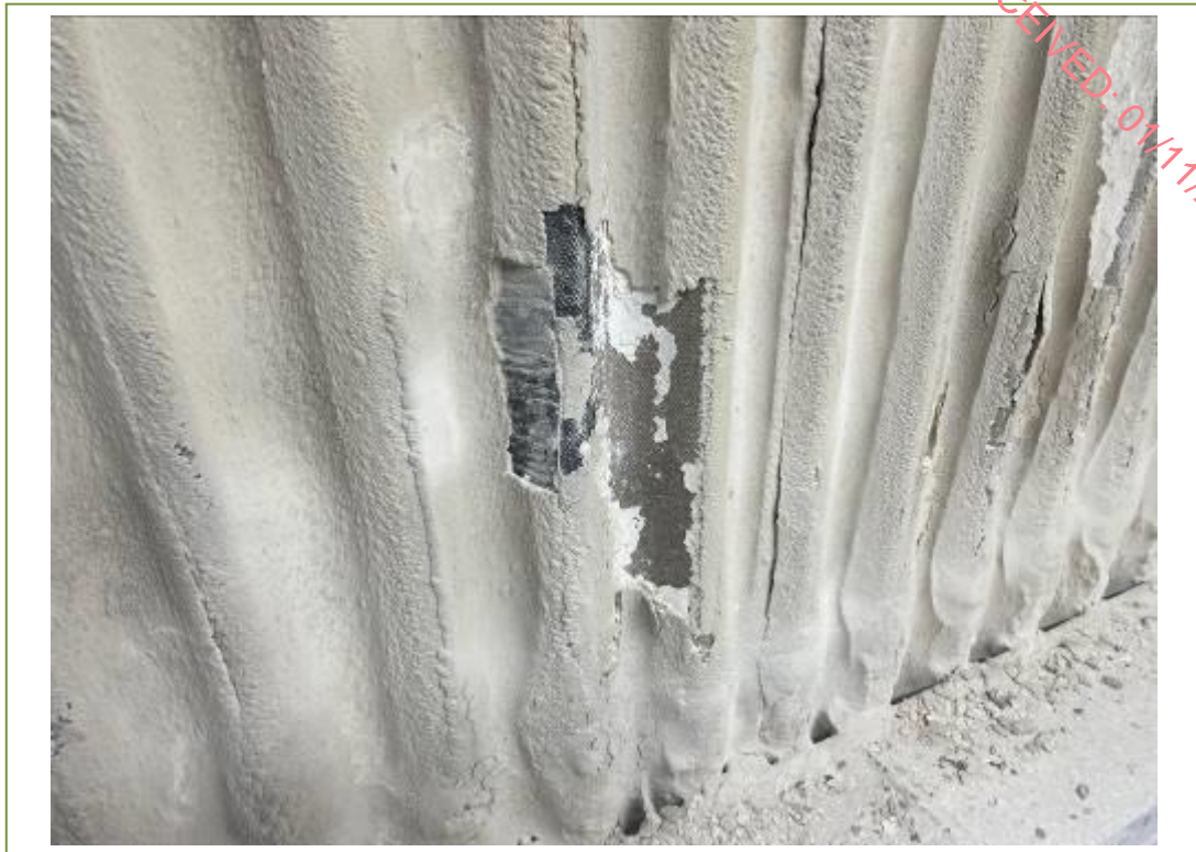
Large buildup of lime dust is firmly adhered to the side sheeting
