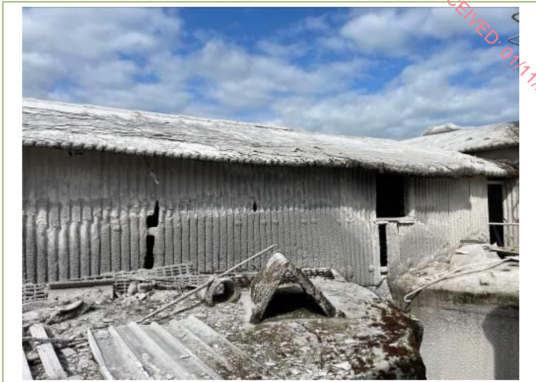
Large amounts of lime dust is visible on the roof and sides of the sheeting
