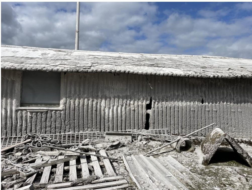
Lime/dust on equipment. ACMs may be concealed underneath
