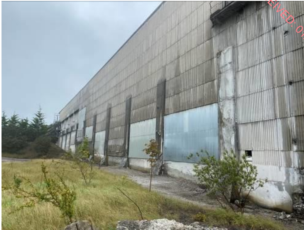
Sections of the asbestos cement cladding on the rear side of the shed have been replaced but a large quantity remains
