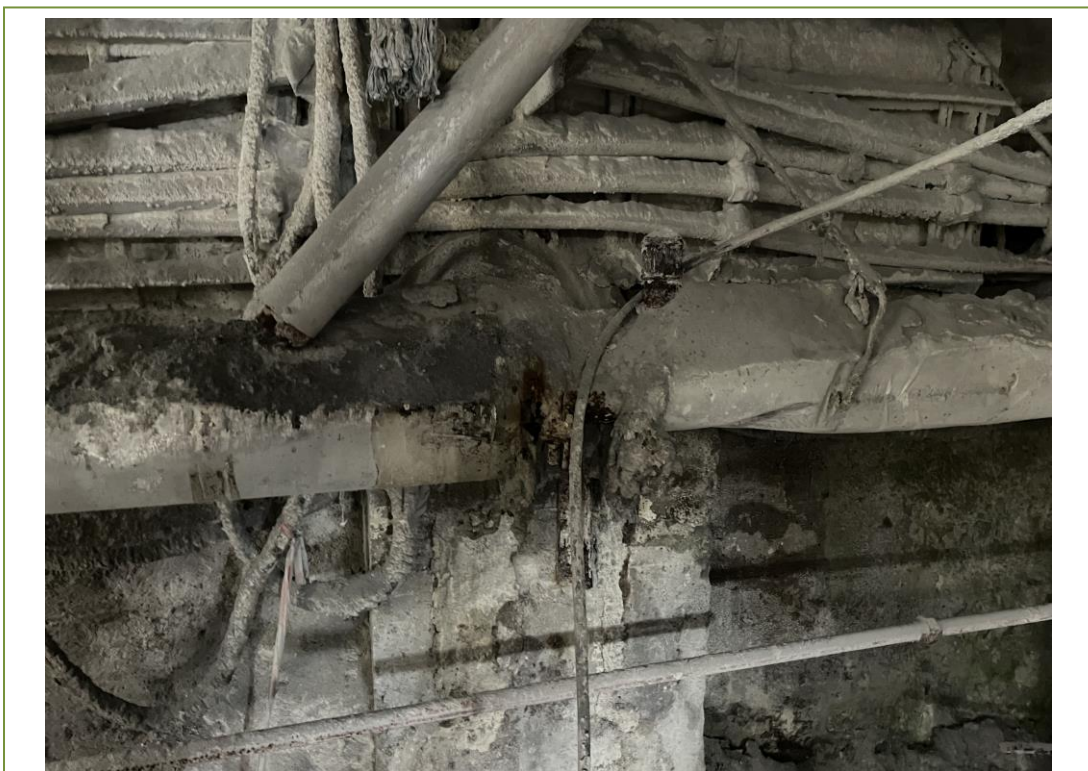
Lime/dust on pipework insulation. ACMs may be concealed underneath
