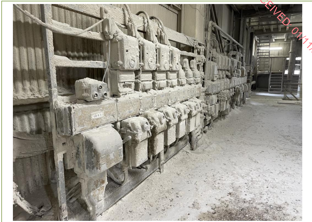
Lime/dust on electrical equipment. ACMs may be concealed underneath
