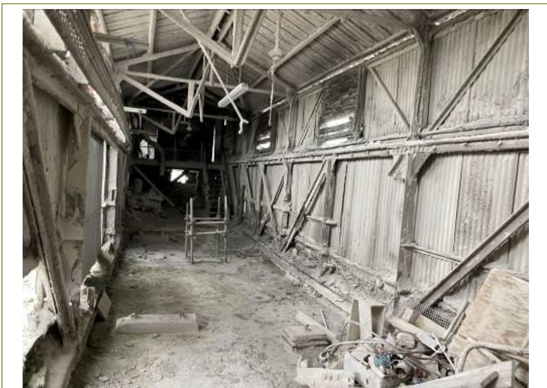
The roof area on some of the walkway is metal but the side sheeting is asbestos cement
