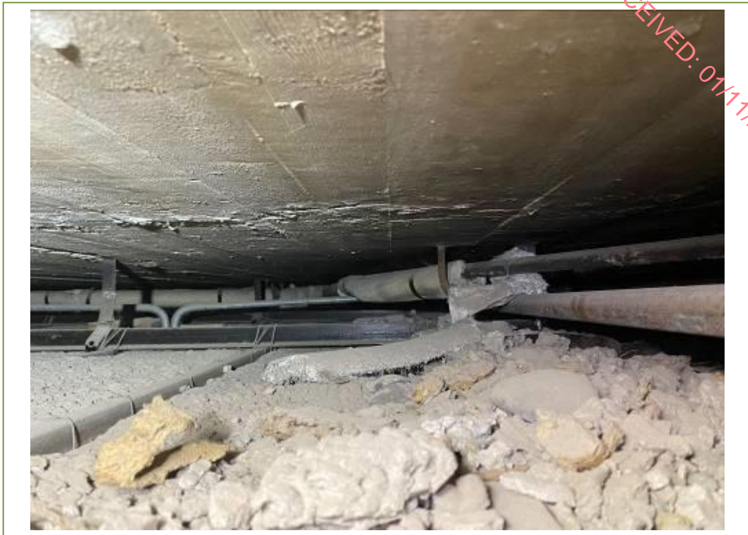
View of the thermal insulation over the original ceiling and 1 st floor
