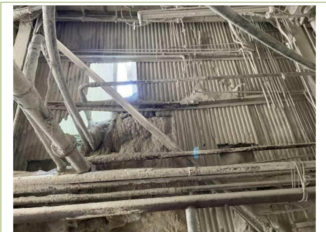
Internal view of the side sheeting showing the level of lime dust on the sheeting
