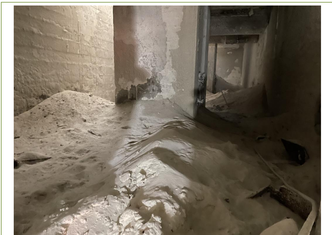
Lime/dust on equipment. ACMs may be concealed underneath
