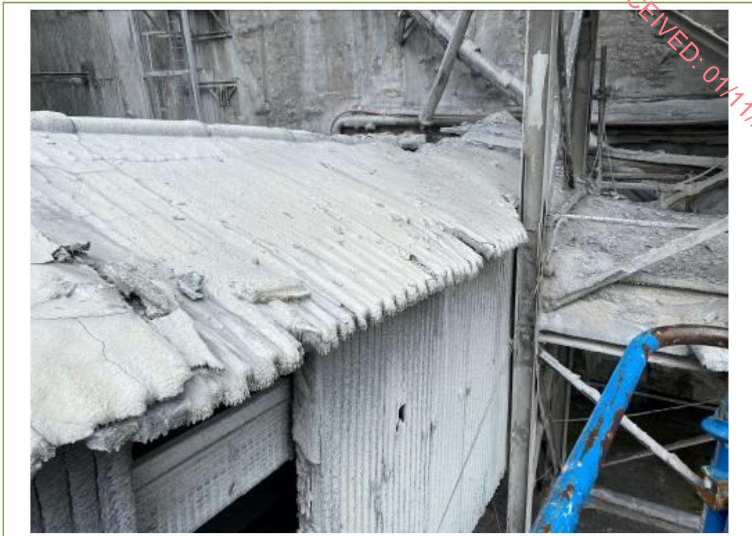
A large amount of lime dust is present on the asbestos cement sheeting
