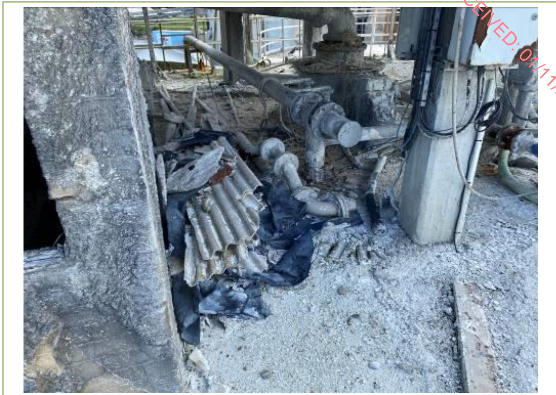
Sheets are damaged and remain on top of the silo from previous removal/cleaning work carried out
