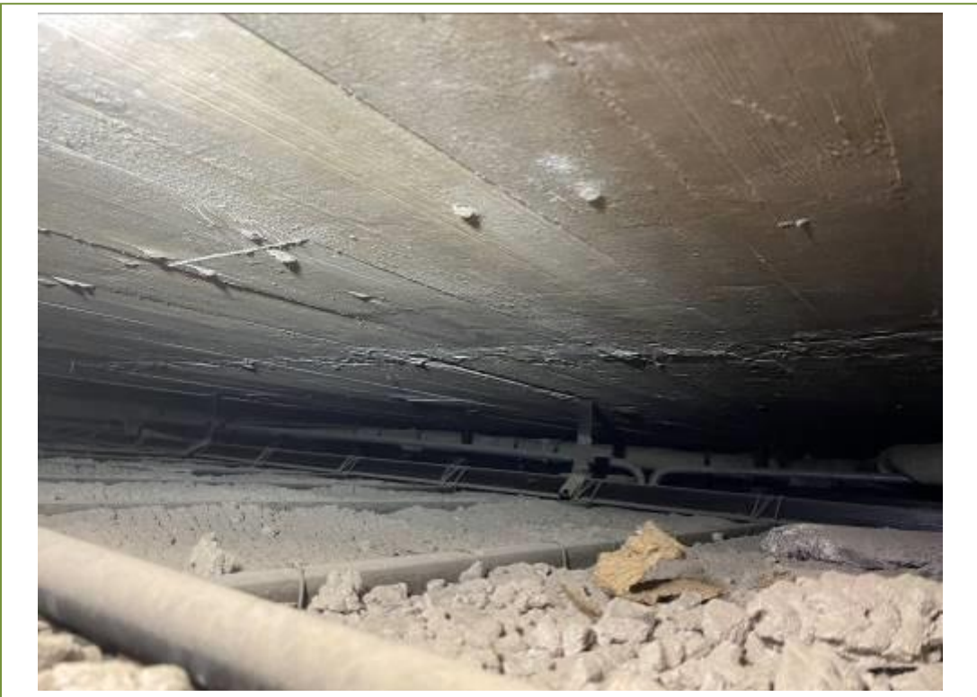
View of the thermal insulation over the original ceiling and 1 st floor
