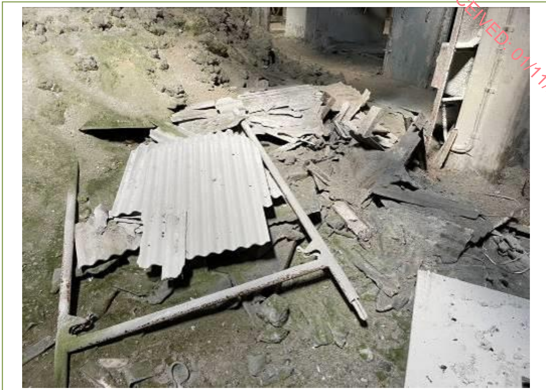
Internal cement sheeting debris
