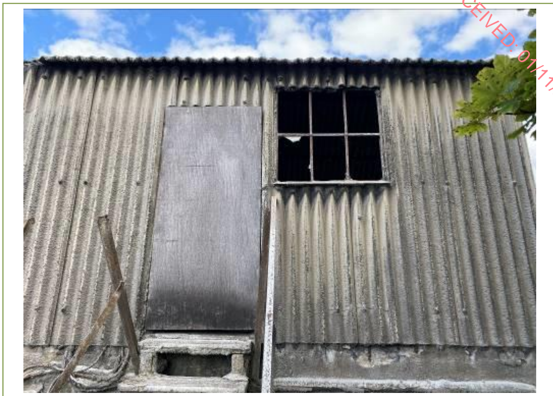
View of the asbestos cement side sheeting
