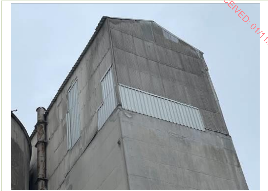
View of the high-level side & gable sheeting on the south side
