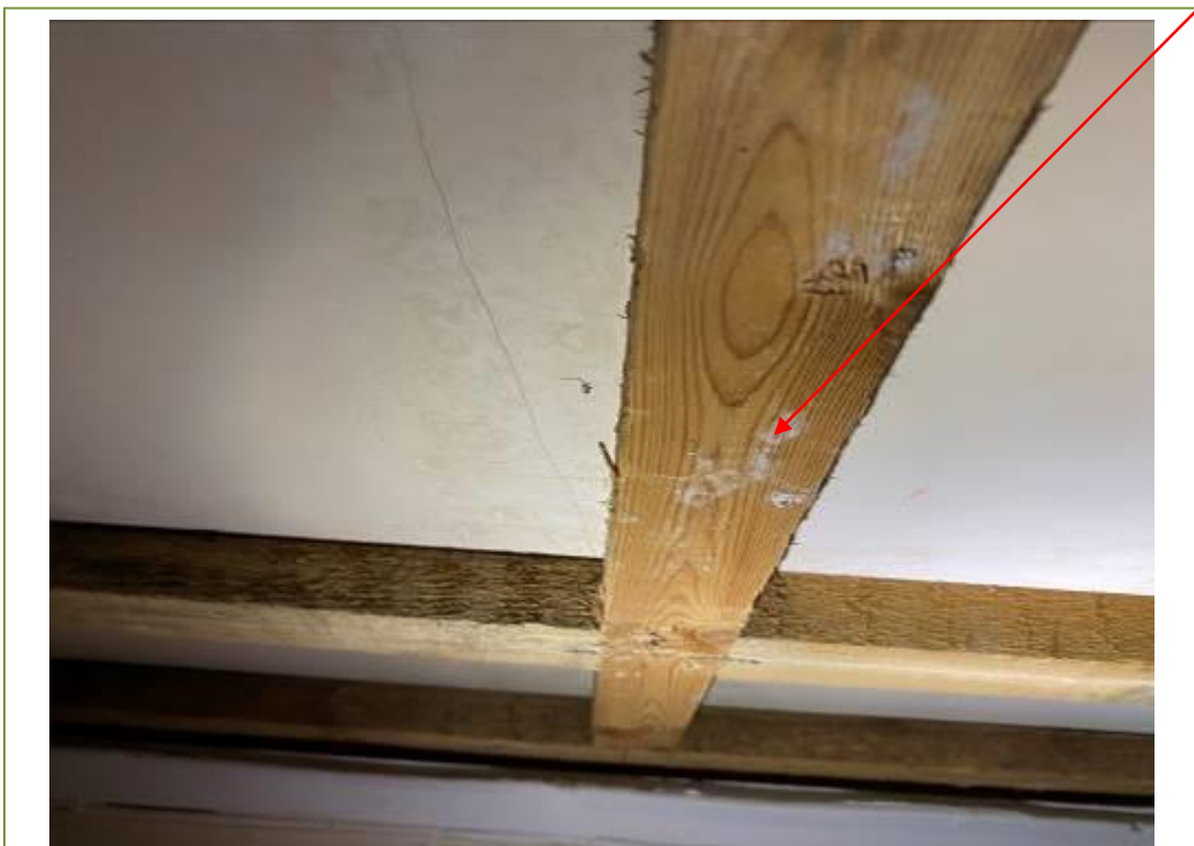
View of the AIB residues remaining on the ceiling tile supports on the 1 st floor hallway
