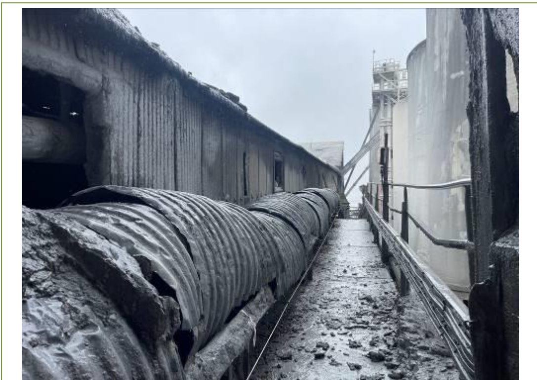
View of the asbestos cement sheeting from the rear walkway
