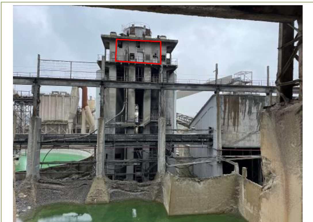
View of asbestos cement sheeting at the rear of the penthouse
