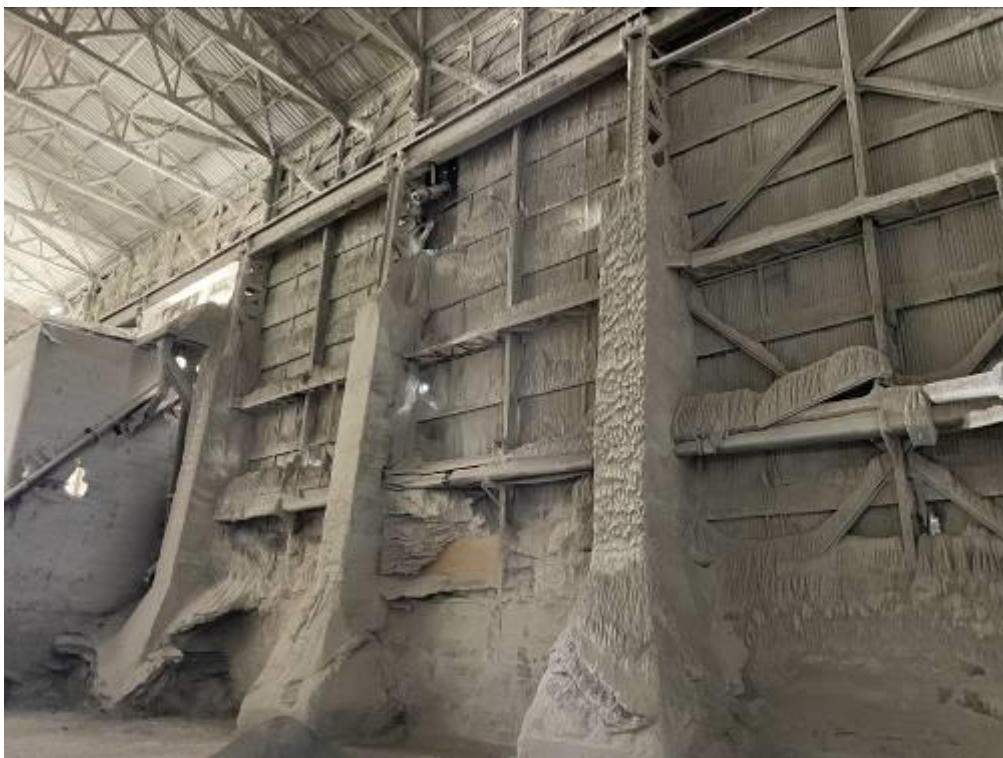
Large deposits of lime dust are adhered to the asbestos cement side sheeting
