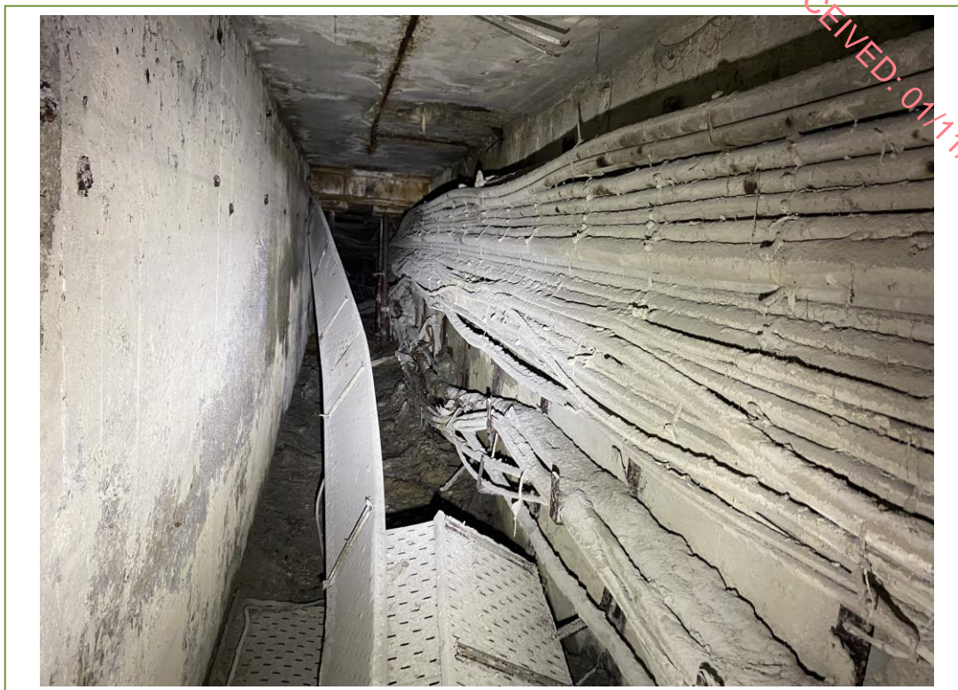
Underground electrical service tunnels. May contain ACMs
