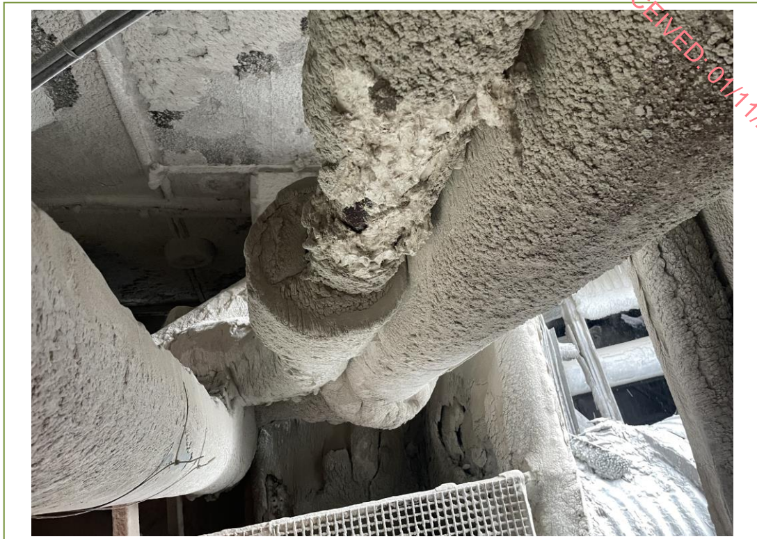
Lime/dust on damaged asbestos pipework insulation
